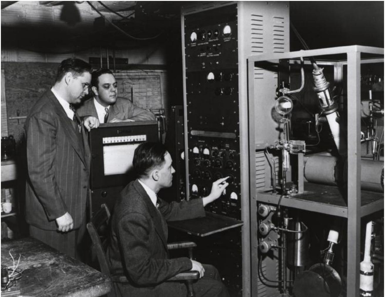
Figure 37. A. O. Nier and two individuals from Consolidated Electrodynamics examining 60° mass spectrometer, which was the prototype for the Consolidated-Nier commercial instrument.
