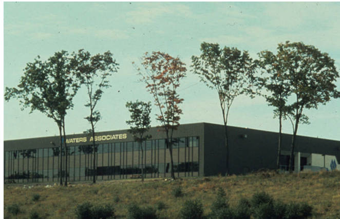
(figure 11) Waters Associates' Milford plant, 1974-1976.
