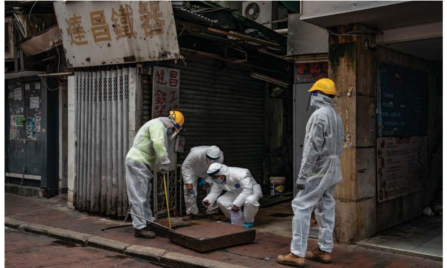
Workers examine a sewer in a Hong Kong neighborhood after a COVID-19 outbreak in the area, January 2021.
